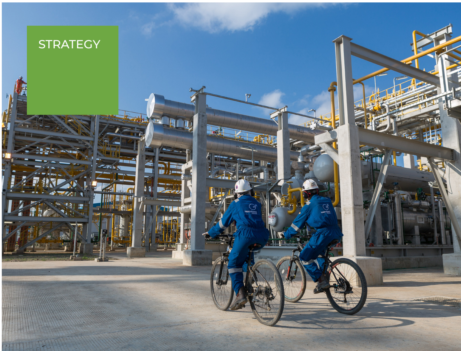
Central Processing Plant, Block A, East Aceh, Indonesia
